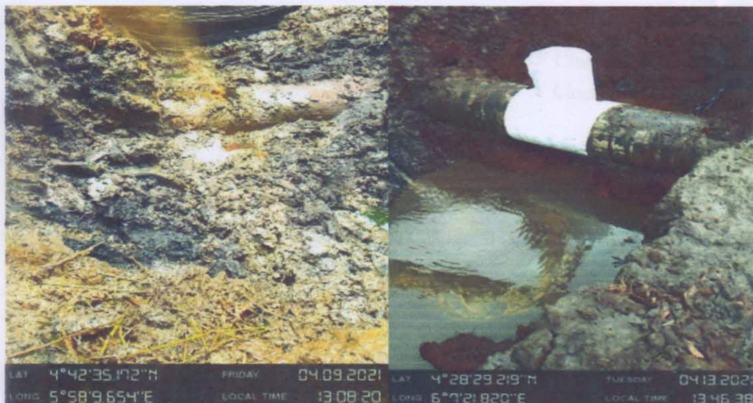
FIG.3 SHOWING 3" VALVE AT 12' O CLOCK
